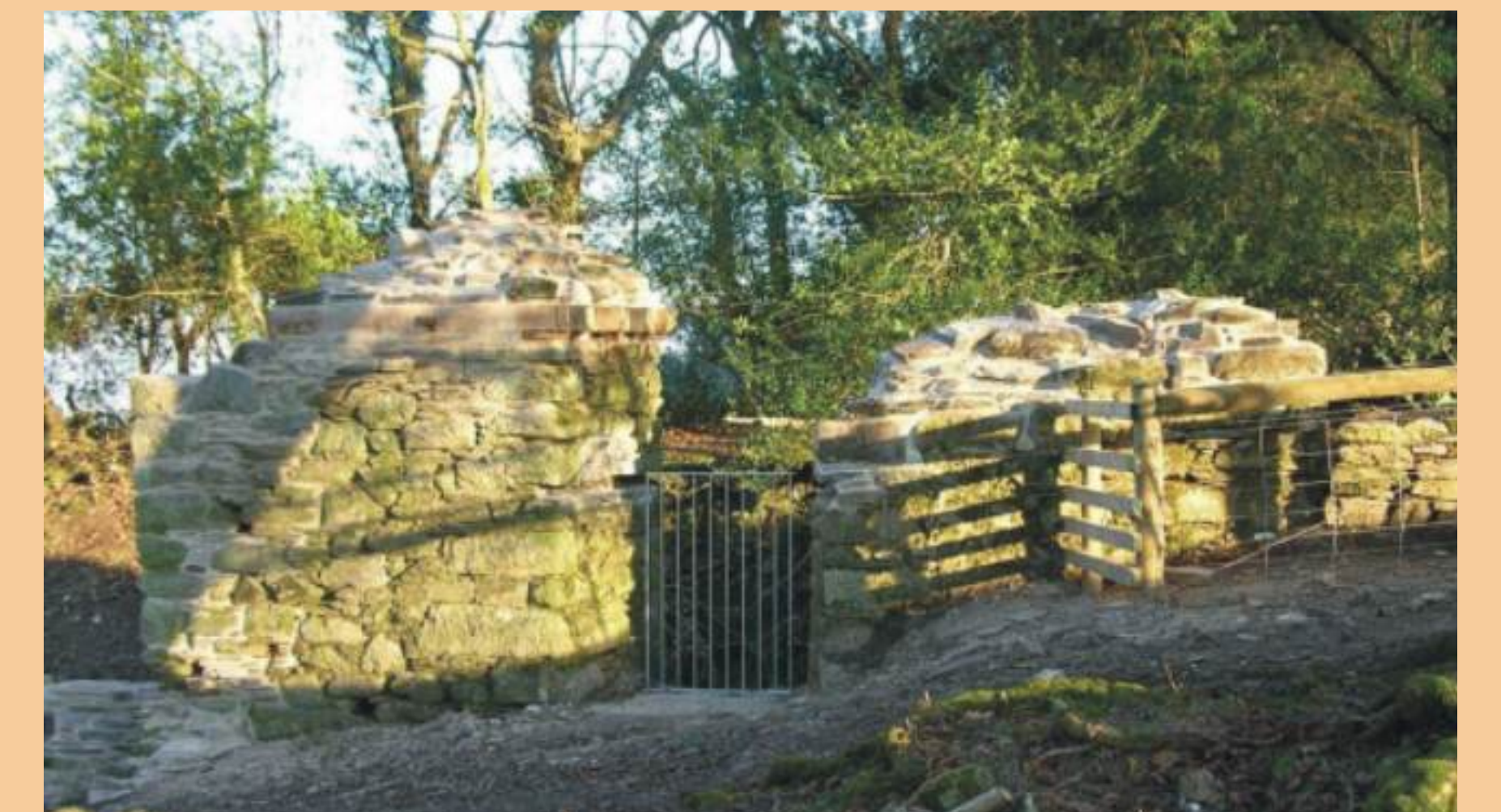
Wheal Tom pumping engine house bob wall
